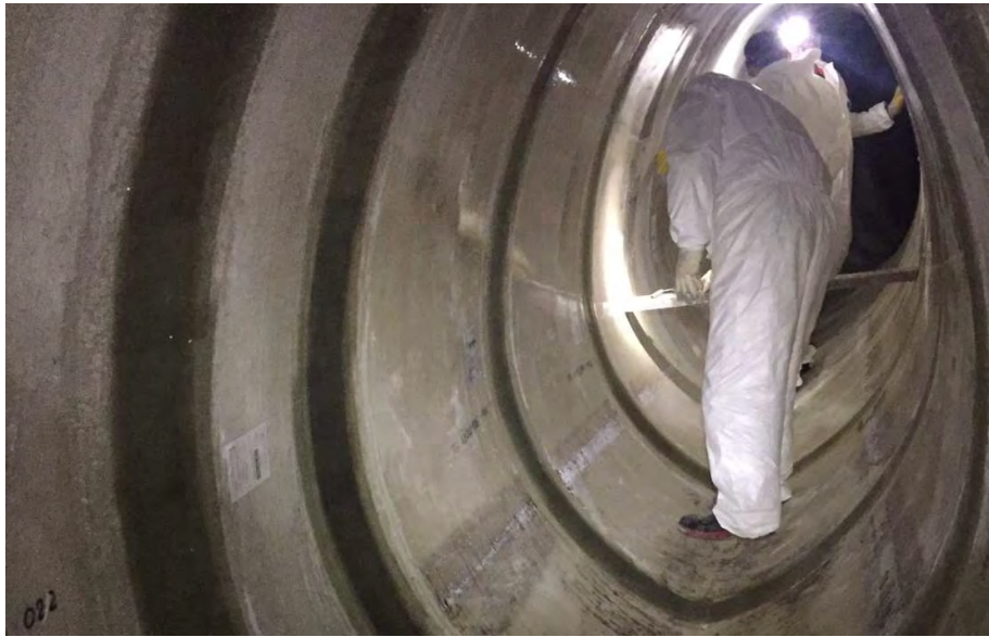
Chamber renovation with the use of basalt tiles
